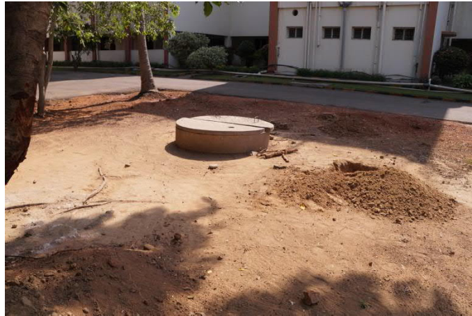
Fig. 7.5: Rain Water Harvesting Pits
