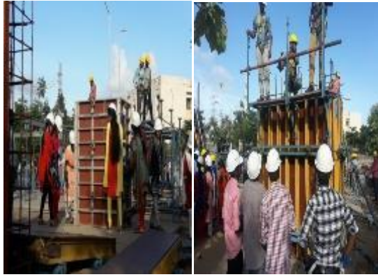
Students undergoing hands on training at L&T Skill training centre, Kanchipuram
